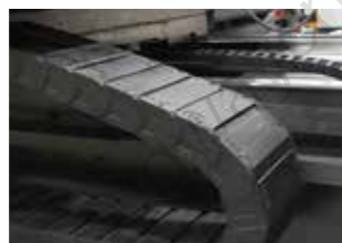
Hidden cabling design
